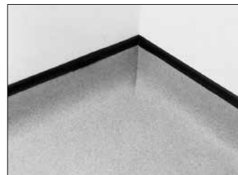
6. Chemical weld to complete the section.
