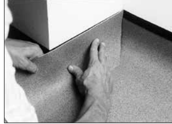
3. Take a separate piece of FiberFlex® and fit to the back of the internal corner.
